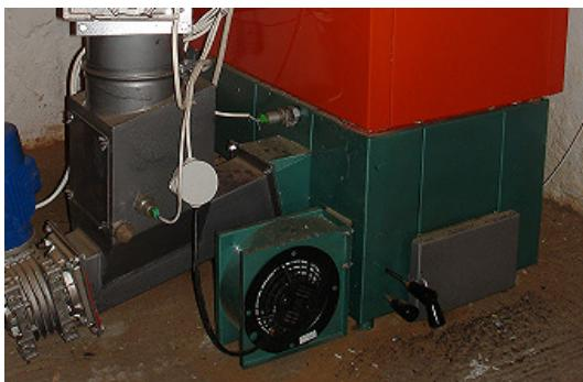
Fig. 3. View of an air distribution box
